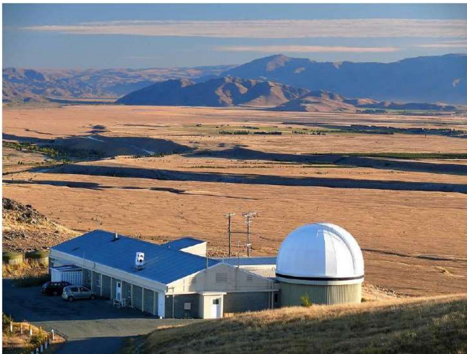
1-m McLellan telescope building at Mt John Observatory
